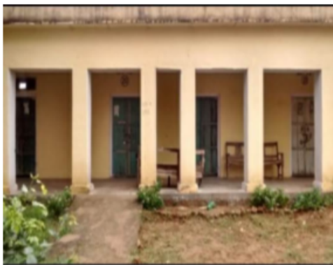
Building Front View
