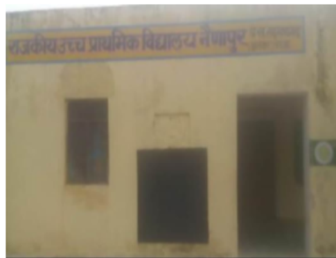
Building Front View
