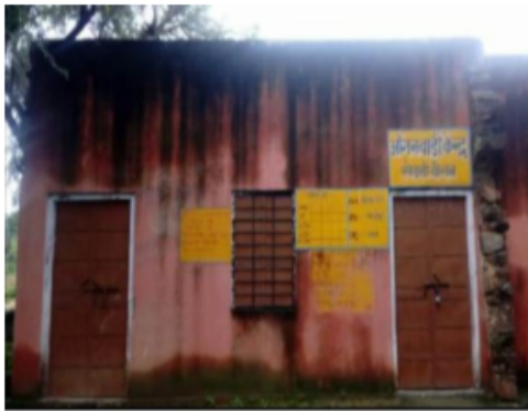
Building Front View
