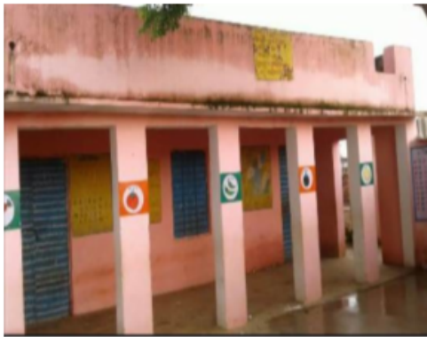
Buildina Front View
