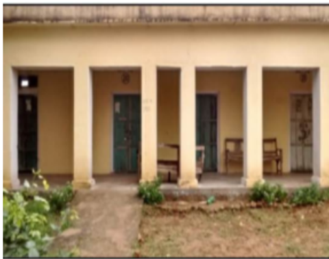
Building Front View
