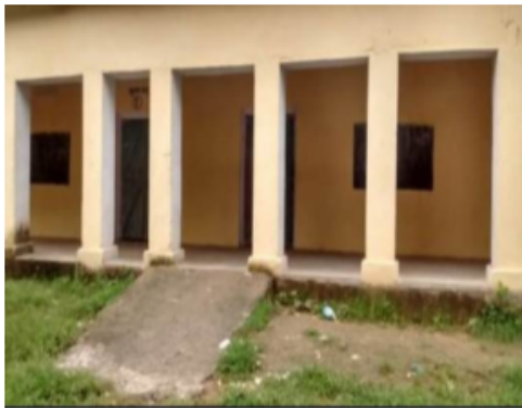
Building Front View
