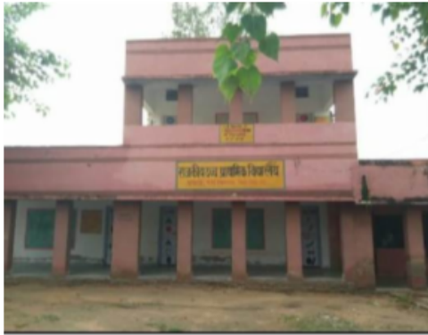
Building Front View
