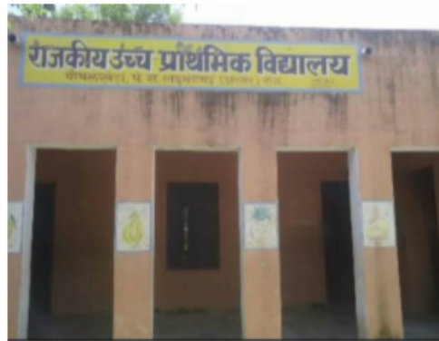
Building Front View
