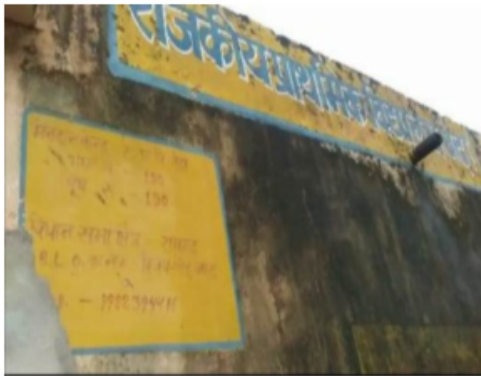
Building Front View
