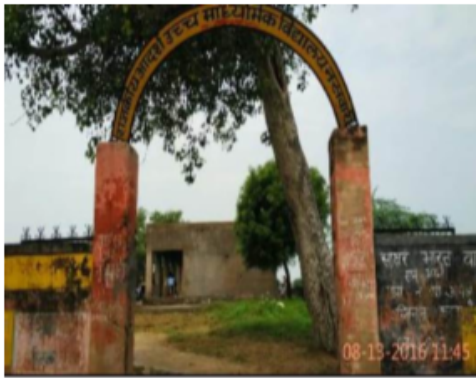
Building Front View
