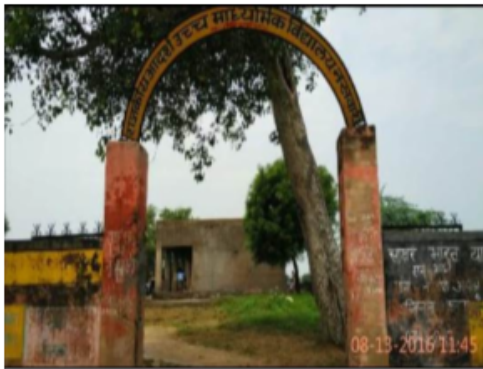
Building Front View
