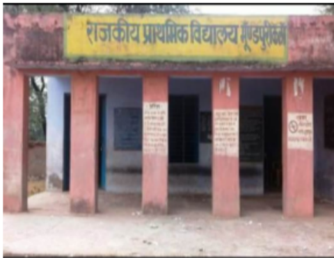
Building Front View
