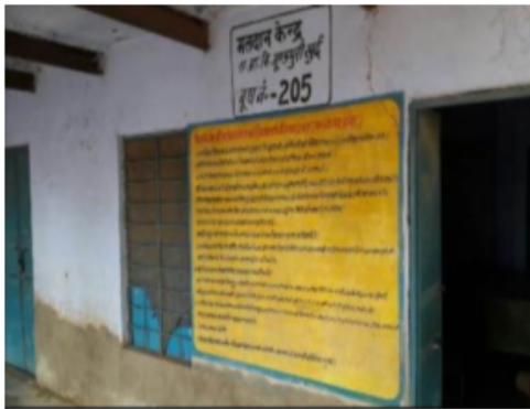
Building Front View
