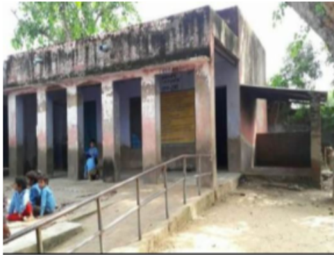
Building Front View
