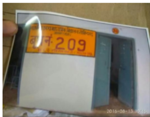
Building Front View
