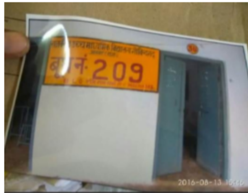
Building Front View
