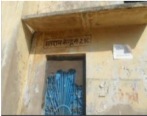
Building Front View
