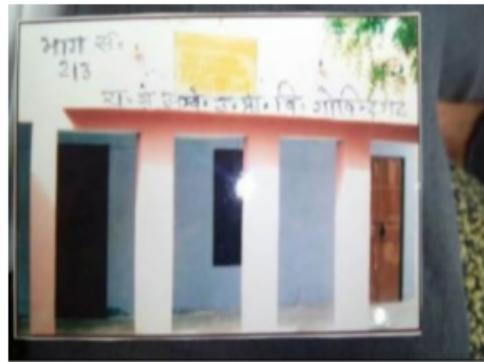
Building Front View
