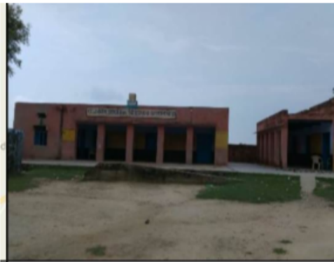
Building Front View
