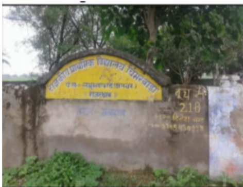
Building Front View
