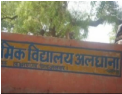
Building Front View
