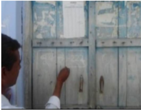
Building Front View
