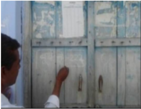
Building Front View
