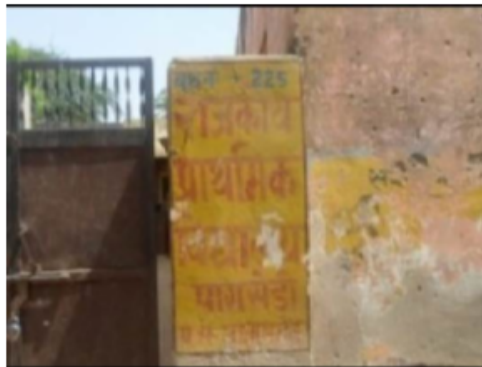
Building Front View
