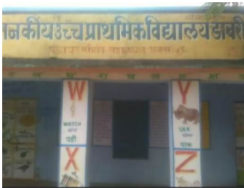
Building Front View
