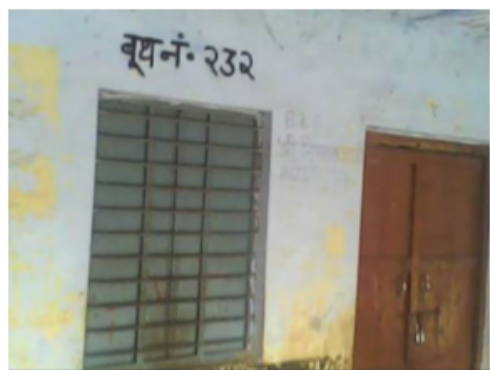
Building Front View
