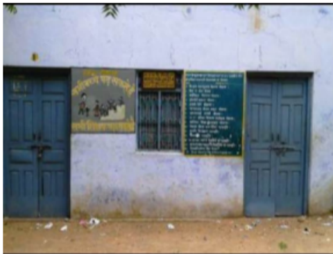
Building Front View
