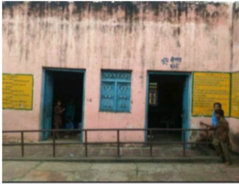
Building Front View
