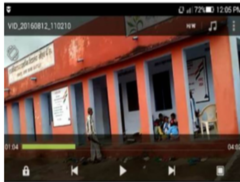
Building Front View
