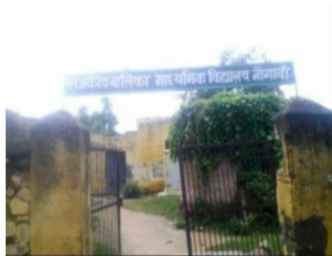
Building Front View
