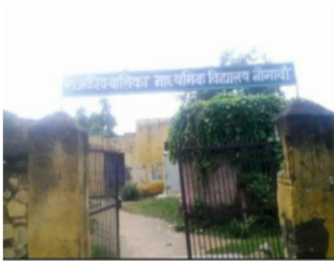
Building Front View
