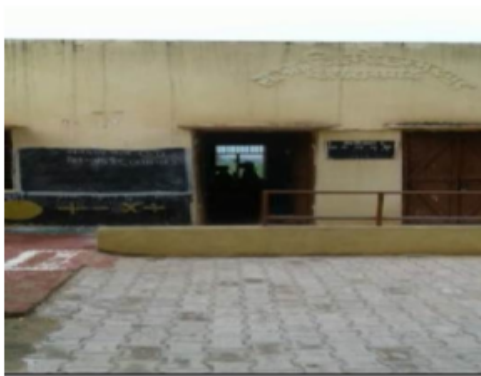
Building Front View
