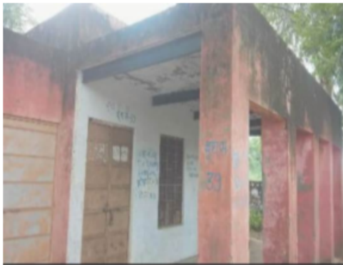
Building Front View
