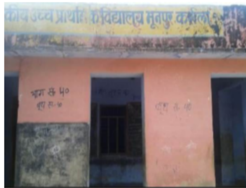
Building Front View
