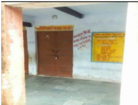
Building Front View
