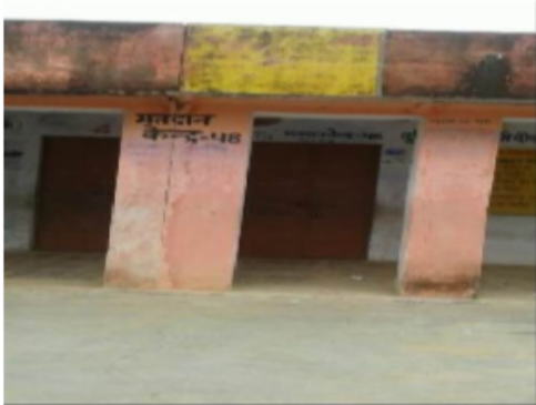
Building Front View
