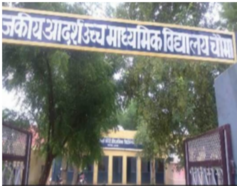
Building Front View
