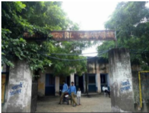
Building Front View
