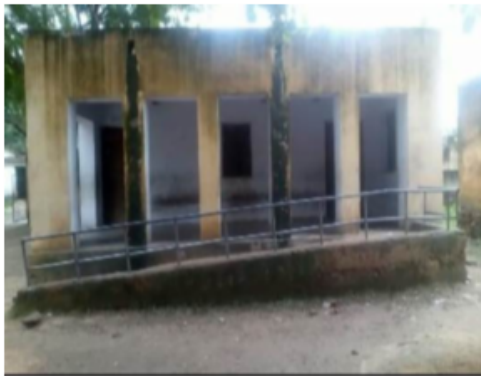
Building Front View
