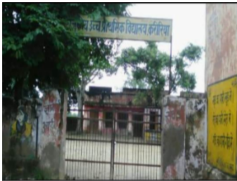
Building Front View
