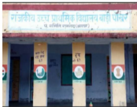
Building Front View
