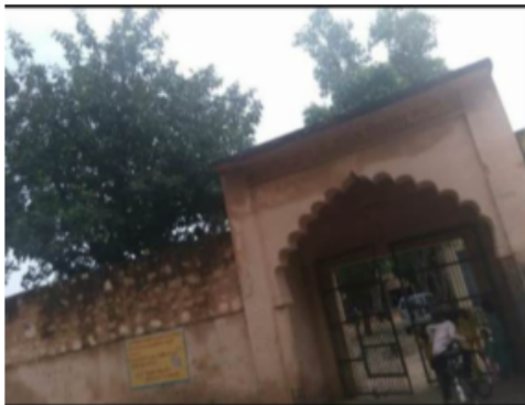
Building Front View
