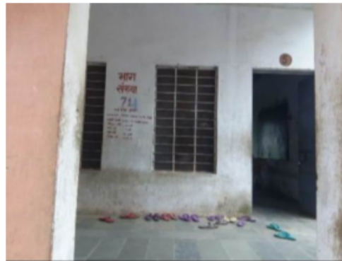
Building Front View
