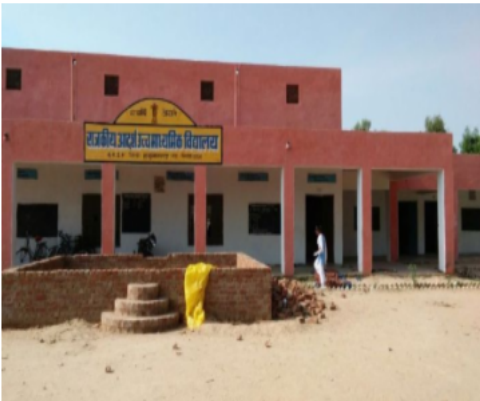
Polling Station Building Front View
