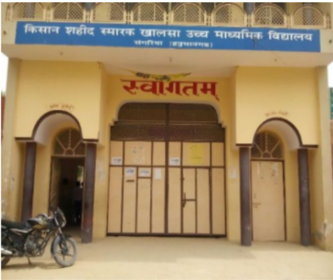
Polling Station Building Front View
