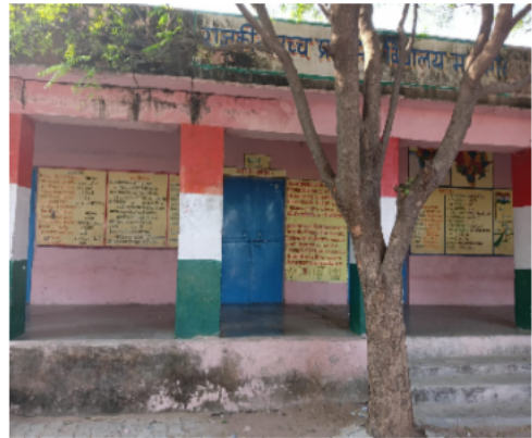
Polling Station Front View
