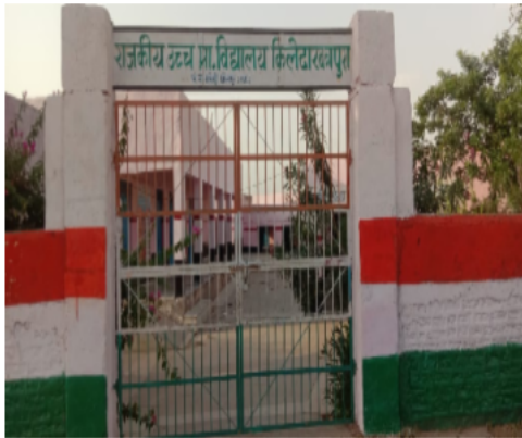
Polling Station Building Front View
