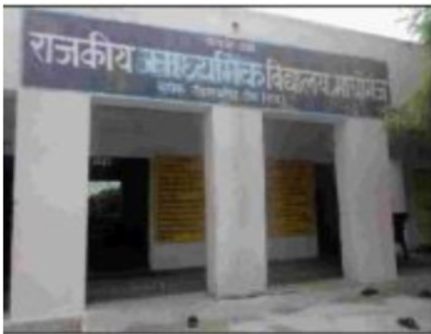
Building Front View
