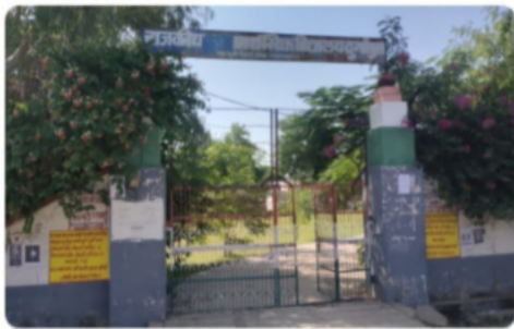
112 Polling Station Building front view
