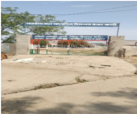
Polling Station Building Front View
